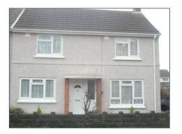
Our team installed a Permaroc insulated over render system with 60mm phenolic insulation and dash render finish. All reveals were insulated and there was particular emphasis on correct detailing to the plinths to ensure no cold bridging and maximum efficiency to all properties.
